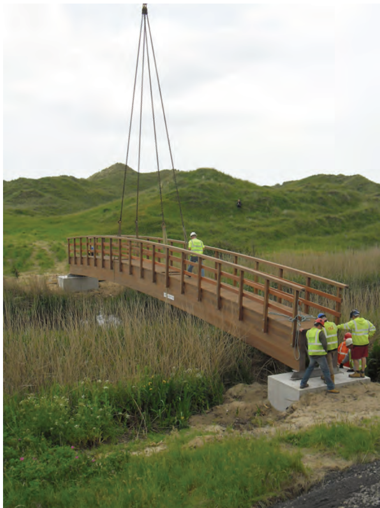
Picture 4.2 Installation of Bridge Linking Neath Port Talbot and Bridgend
